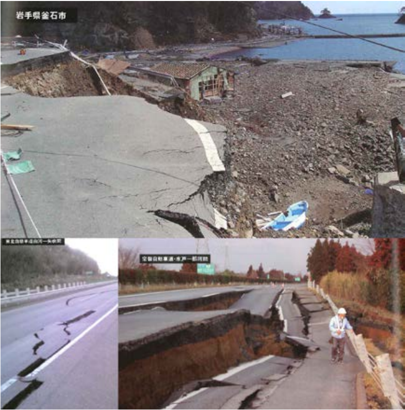
Fig. 1. Road damaged by 3.11 earthquake
